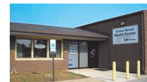
Blackhawk Park School-Linked Health Center 330 15th Avenue Rockford, IL 61104
